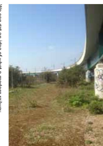
We can get an idea of what a modern railway viaduct will look like from this image of the recently constructed Hitchin Flyover!
